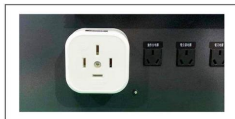
Power supply socket
