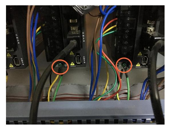
Connect a cable from driver GND to COM2 connector on 5/12V power supply(in the electricity box, there are three power supplies, 5/12V is the middle one)
